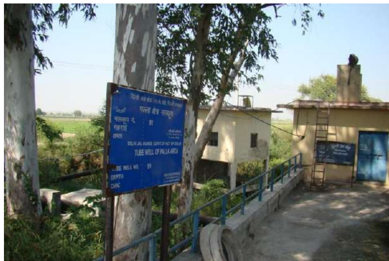
Pic 4: Ranney and tube well of DJB in flood plain
