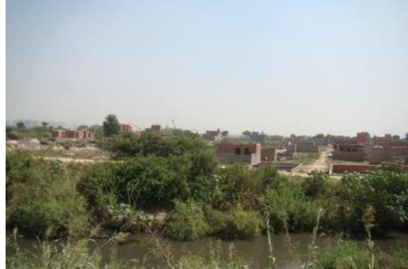
Pic 24: Construction in flood plain across Ali Drain
